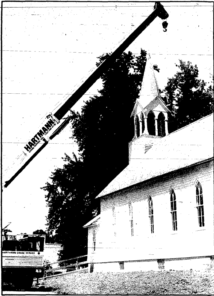
PAINTER MIKE ENCONTRO of Omaha dangles nearly 55 feet above the ground as he paints the steeple of the Winside Theophilus Church Museum. Encontro is pictured sitting in a chair hooked to the end of a cable operated by Owen (Tuffy) Hartmann, owner of Hartmann Crane Service of Winside.
